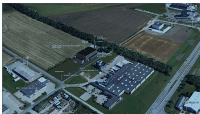
GTS Test Center (forslag) – Gas substation - Cocio
